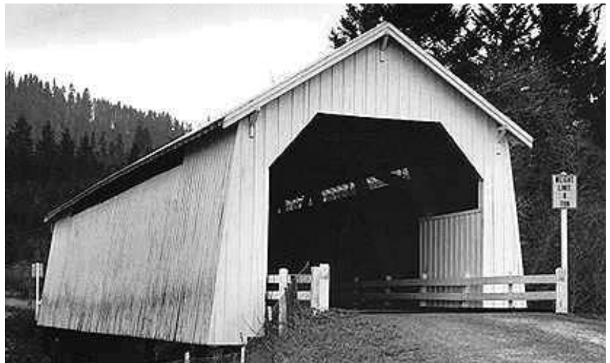
Hayden Bridge, Benton County
